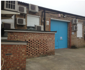
Large door on the side of 714
