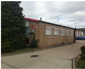
714 Banbury Avenue from the road
